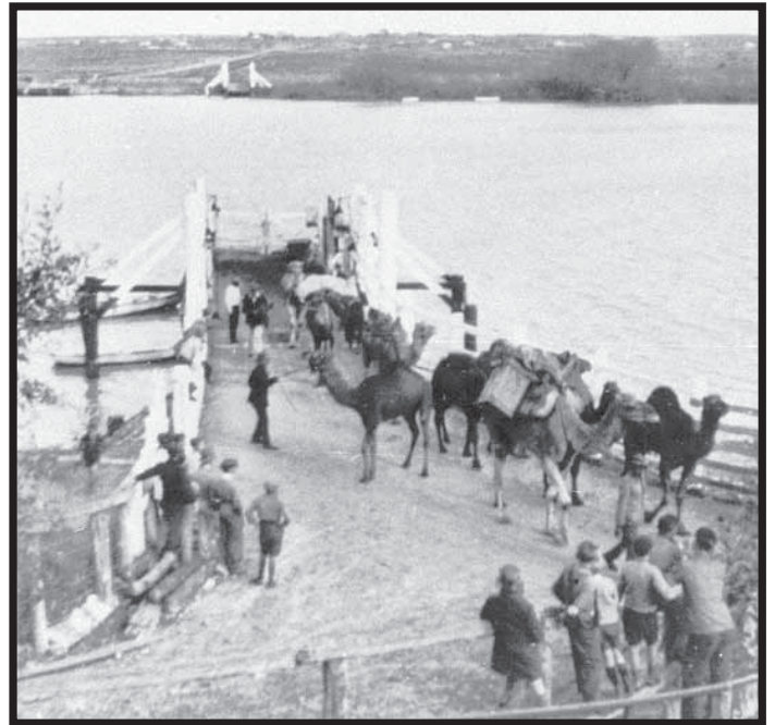
ABOVE: Old TB Ferry.
